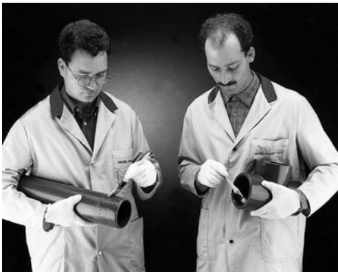
Fig. 7: Applying the cement (sizes d 110 mm and above)
