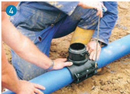
Connection to the plastic pipeline vertically or laterally. Full range of fittings which satisfy all requirements.
