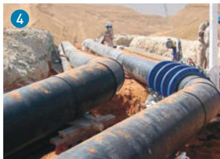
**Variety of connection needs.** Butt-fused segmented fittings can be customised to meet local requirements.
