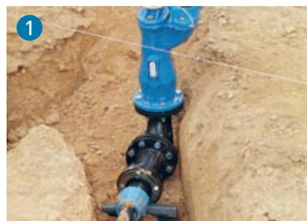
**Easy connection to hydrants.** Transitions between PE lines and metal hydrants are easy and safe to install.
