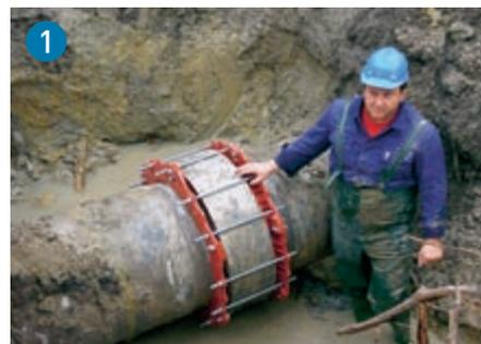
**Repair of leaking joints under pressure.** WAL/V leak clamps provide a dependable repair solution.
