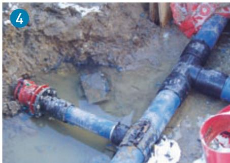
Wide-range fittings for reliable transitions. MULTI/JOINT 3000 offers end-load resistance, without thrust blocks.
