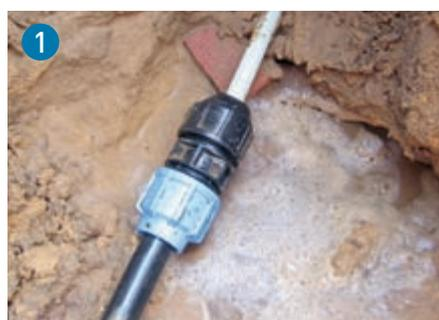
**Easy house connections.** The universal fitting for connecting metric PE pipes to plastic or metal pipes in every situation.
