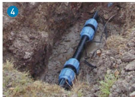
**Simple installation technology.** PE branch-off on an asbestos cement pipe with the MULTI/JOINT wide range coupling.
